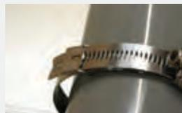
3. Push any remaining band into the buckle for a safe, tidy finish.
