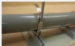
2. Screw the band through the housing using the driver or power tool.
